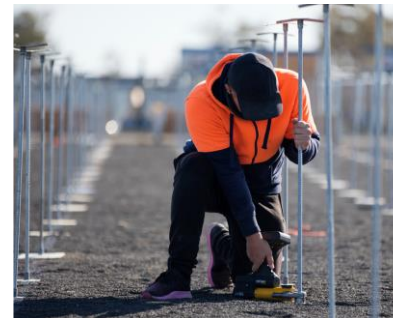
Crimping of bottom plate*
