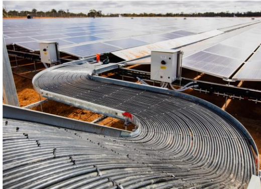
Cable routing (No DC trenching)
