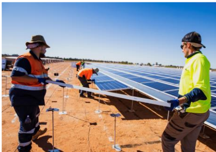
Installation of modules
