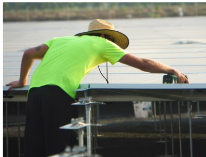
Installation of module clips
