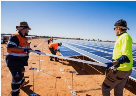
Installation of modules
