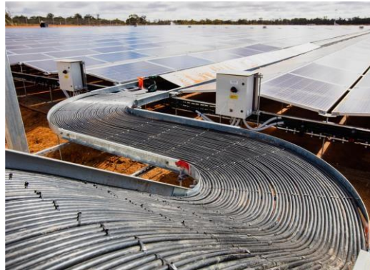
Cable routing (No DC trenching)
