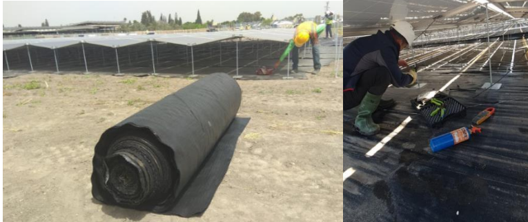
Fabric sheet under the PEG
