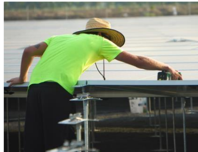
Installation of module clips
