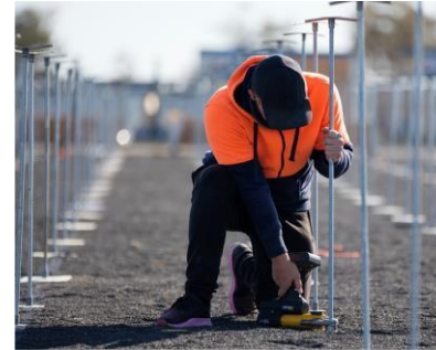
Crimping of bottom plate*
